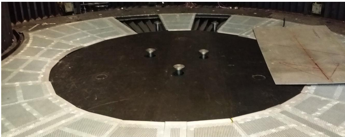
Figure 11. Raised hard points in floor of Space Simulator.
