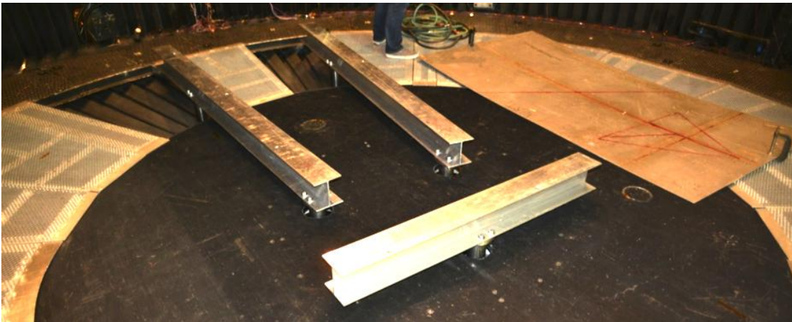
Figure 12. Aluminum I-beams bolted to hard points in chamber floor.
