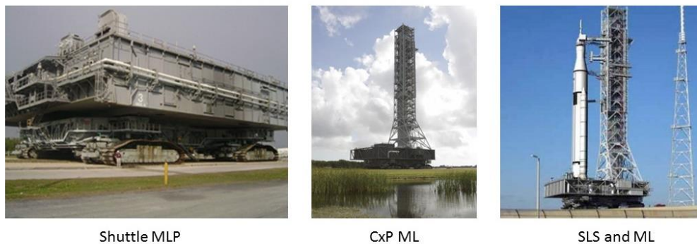
Figure 6. Space Shuttle, Constellation, and Space Launch System Launch Platforms
