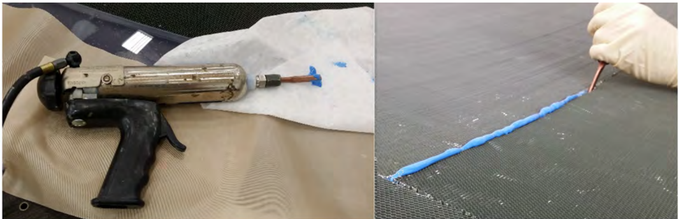
Figure 86. Paste core splice adhesive injection.
