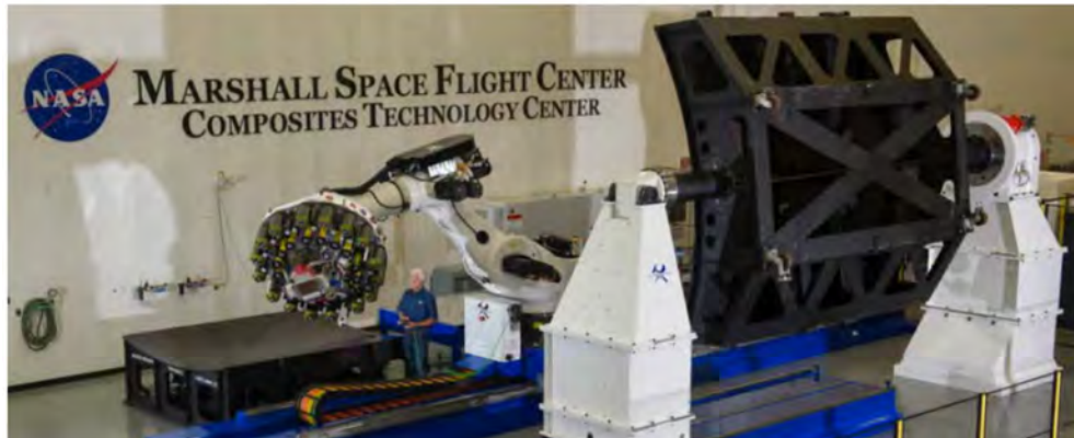
Figure 78. CEUS tool installed in MSFC AFP cell.
