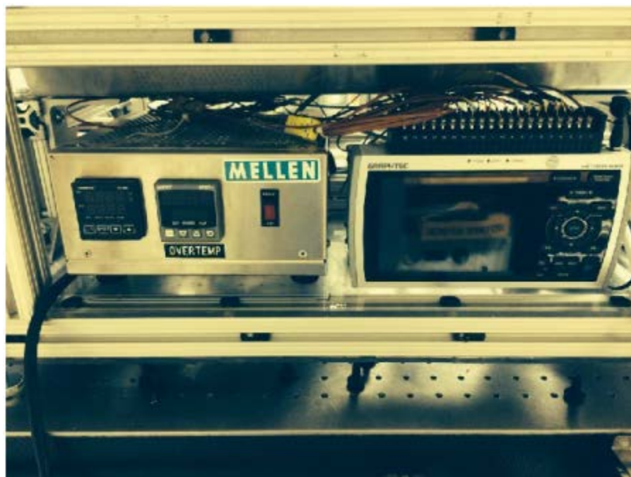
Figure 40.—Furnace Controller and Data Acquisition System.
