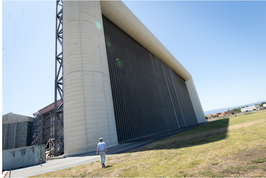
Figure 9. The 80- by 120-Foot Wind Tunnel Inlet. 4
