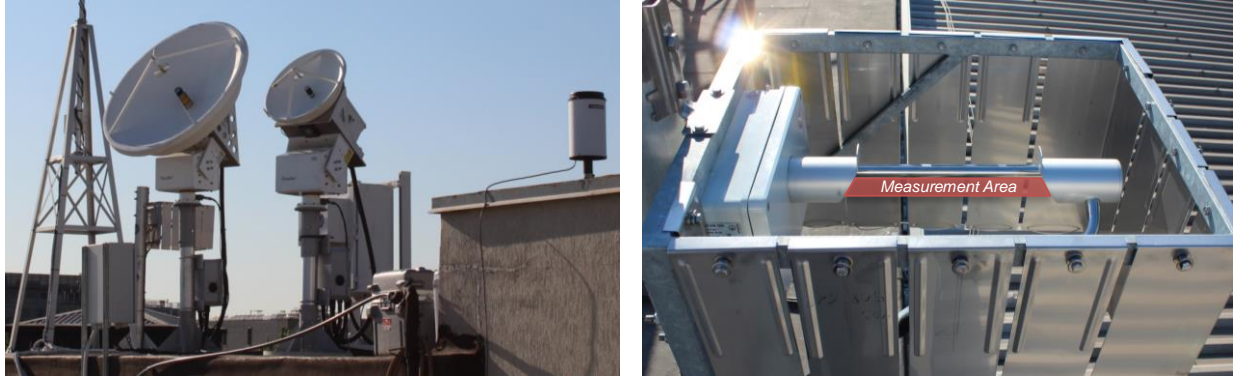
Figure 1. The Ka- and Q-band beacon receivers (left) and the Thies Clima optical disdrometer (right), installed in April 2014 at the POLIMI campus in Milan, Italy.
