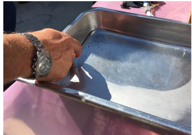
Particulate and Oily Contamination removed from the LOX piping during the Solstice PF Spray Field Cleaning Test
