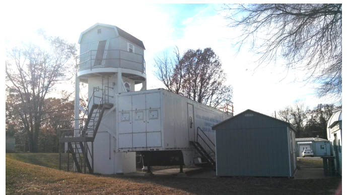
Figure 16. SAS Tower Test Facility (TTF) with Protective Shed on Top of Tower, New Work Shed on Ground and Re-purposed EMC Test Van
