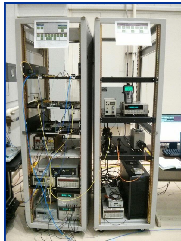
RF/Optical Transmitter and Optical Receiver
