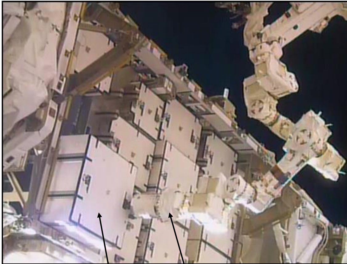
Li-Ion Battery ORU
