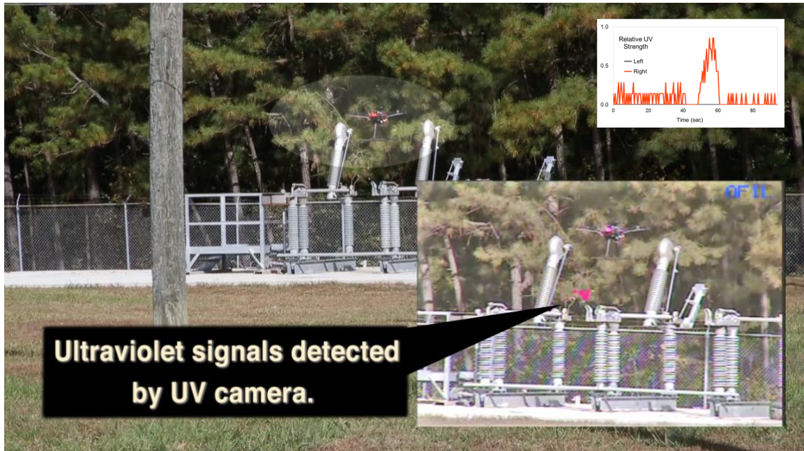
Figure 6. Validation of the compact UV sensor signal with corona camera in a substation measurement flight. The visible camera image shows the UAV above the substation structure (background; UAV is in lightened ellipse). The inset at top right shows the compact UV sensor recording, which reaches a maximum as the UAV passes the corona generator. The inset at bottom right shows the corona camera record; the bright red blobs at the center of the image are locations of UV emission.
