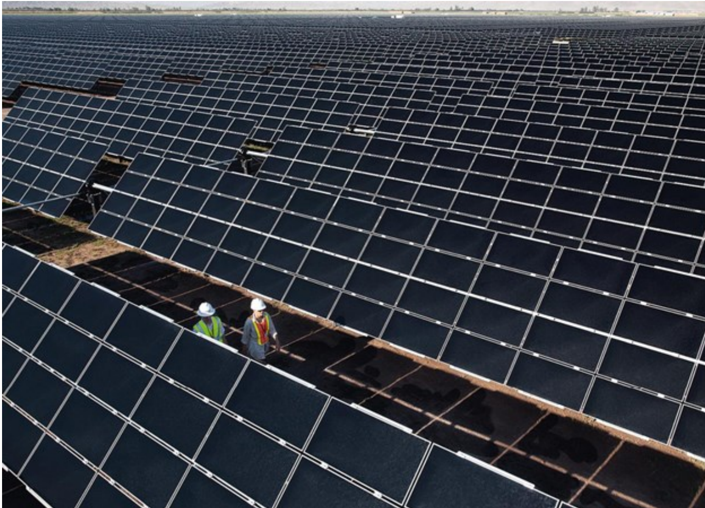
Mount Signal Solar, Imperial County, CA 265 MW, 1980 acres, Largest single-axis tracker
