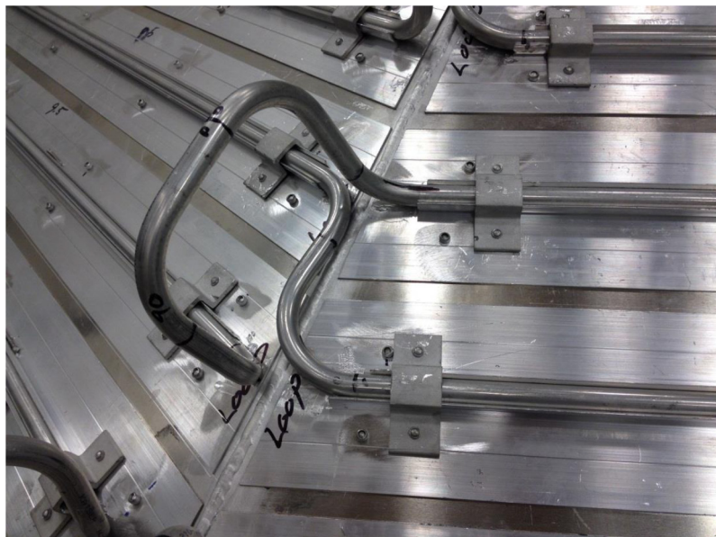
Figure 8. Tubing bent and installed in extruded channels.
