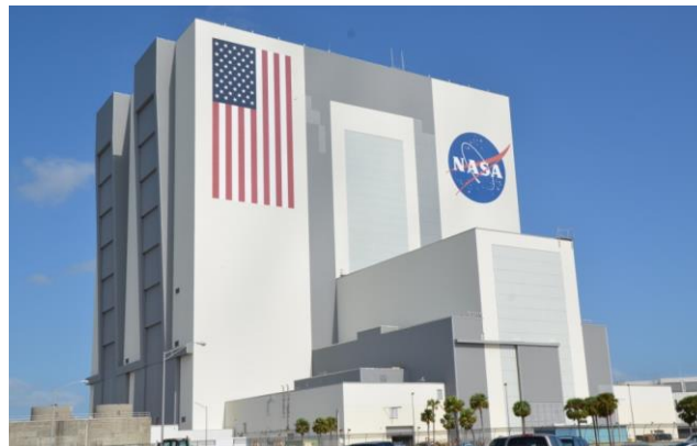
Figure 7-8. Vehicle Assembly Building (VAB)
