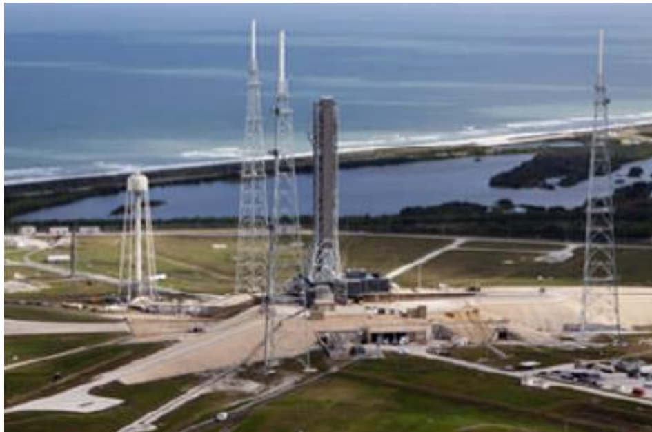
Figure 7-12. Launch Complex 39B (LC-39B)
