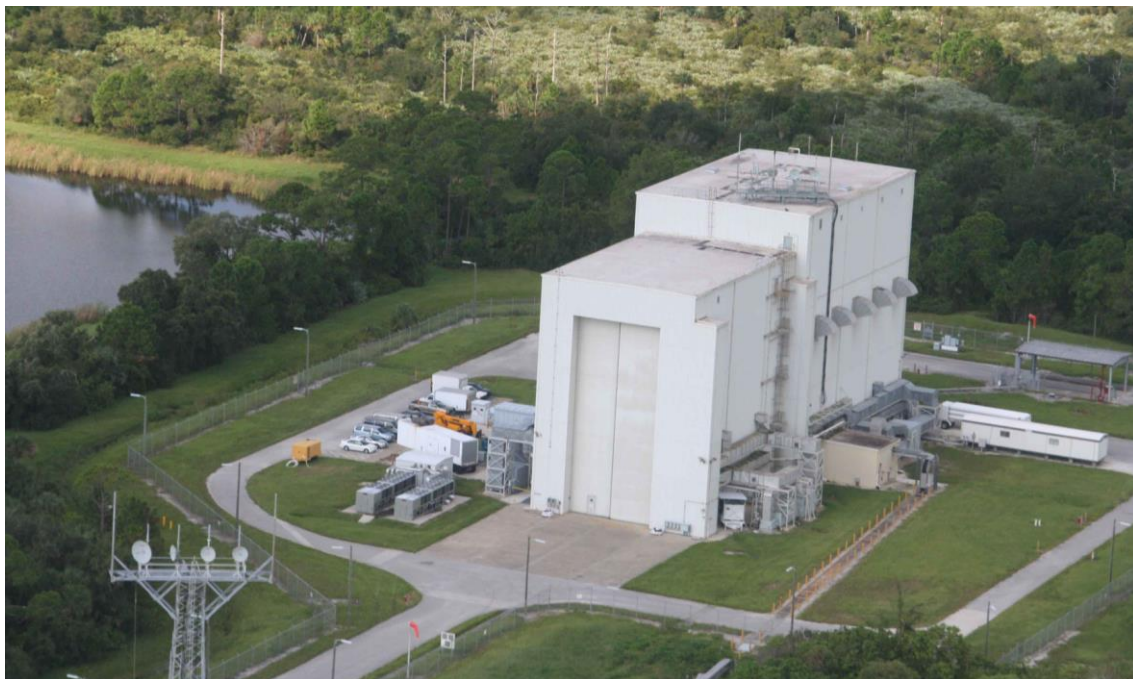
Figure 7-6. Payload Hazardous Servicing Facility (PHSF)
