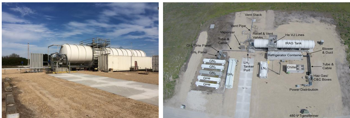
Figure 1. GODU-LH 2 Test Site: Ground Level View (Left); Overhead View (Right)
