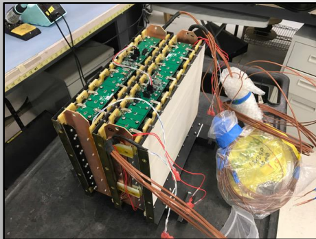
X-57 Thermal Runaway Unit (2 Trays; ½ Module)
