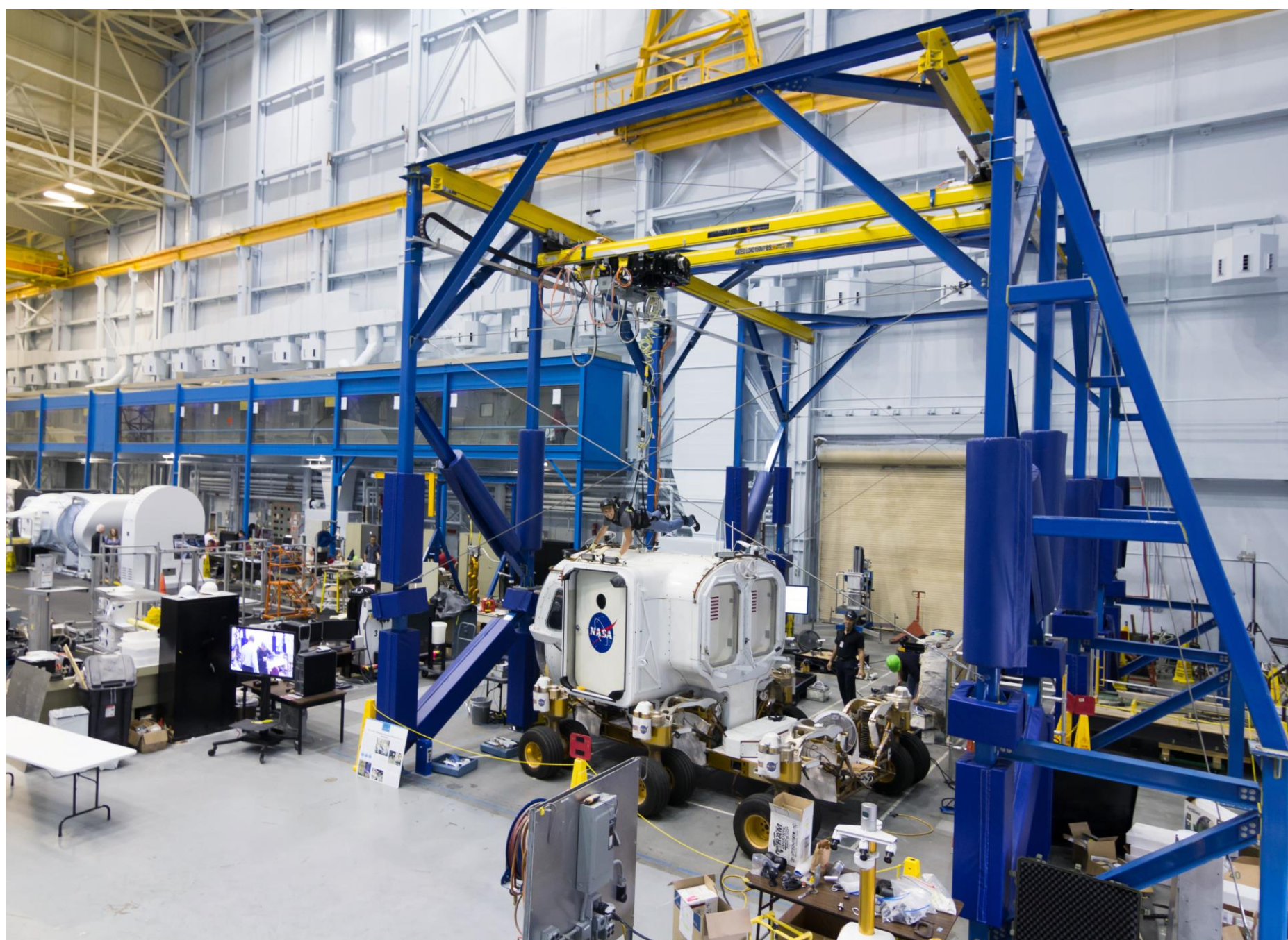
Active Response Gravity Offload System (ARGOS) at JSC
