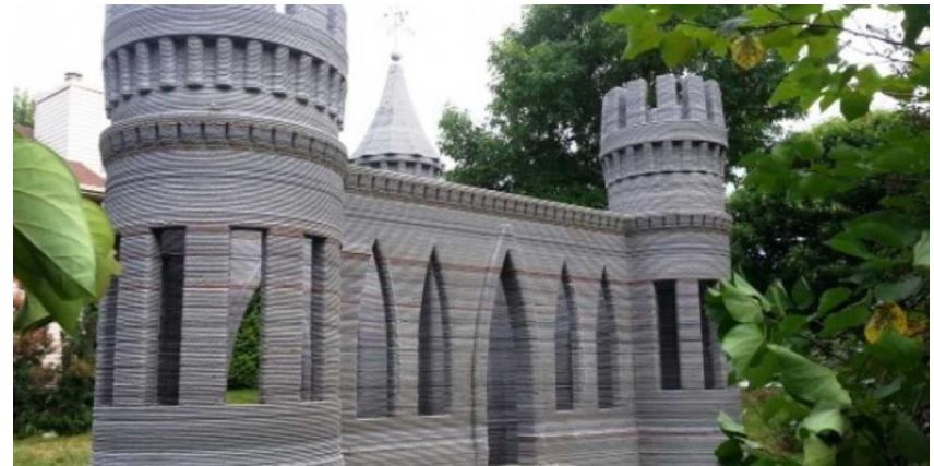
3D printed concrete castle
