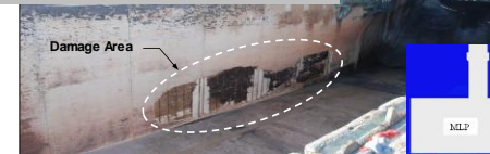
KSC Pad 39A Flame Trench Damage
