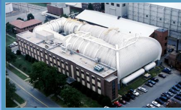
LaRC Transonic Dynamics Tunnel Aeroelasticity & Flutter
