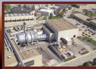
GRC Propulsion Systems Laboratory Engine (and icing) Simulation at Altitude
