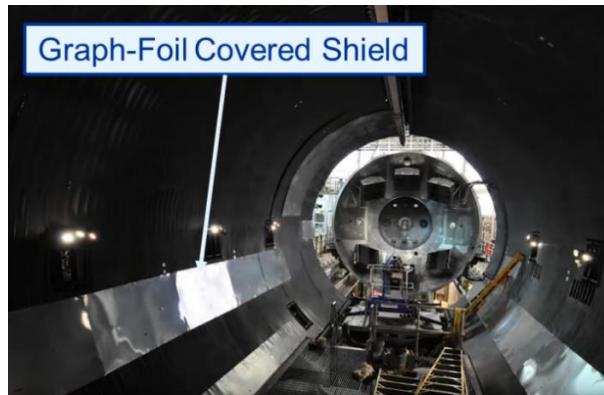
Figure 4. VF-6 during installation of Grafoil® shielding.
