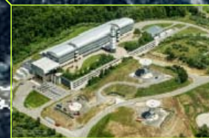
Consolidated Backup, Fairmont WV
