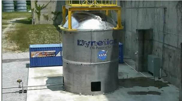
Fig. 30. Moment of burst (note fluid escaping through crack in top dome).
