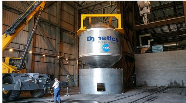
Fig. 23. Integrating the tank and test stand in Iuka, MS.
