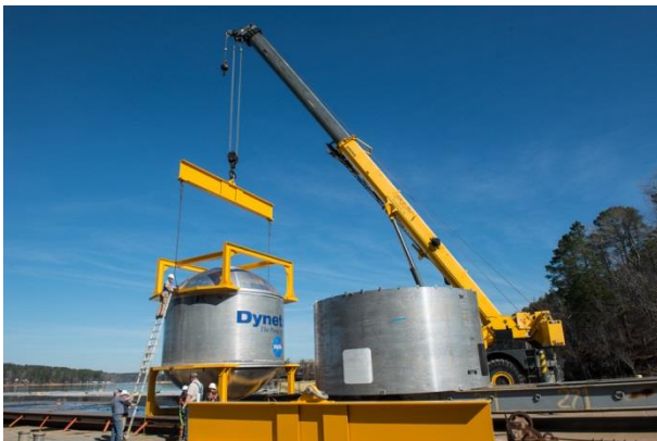
Fig. 22. Placing the tank and fixtures on the barge for transport.
