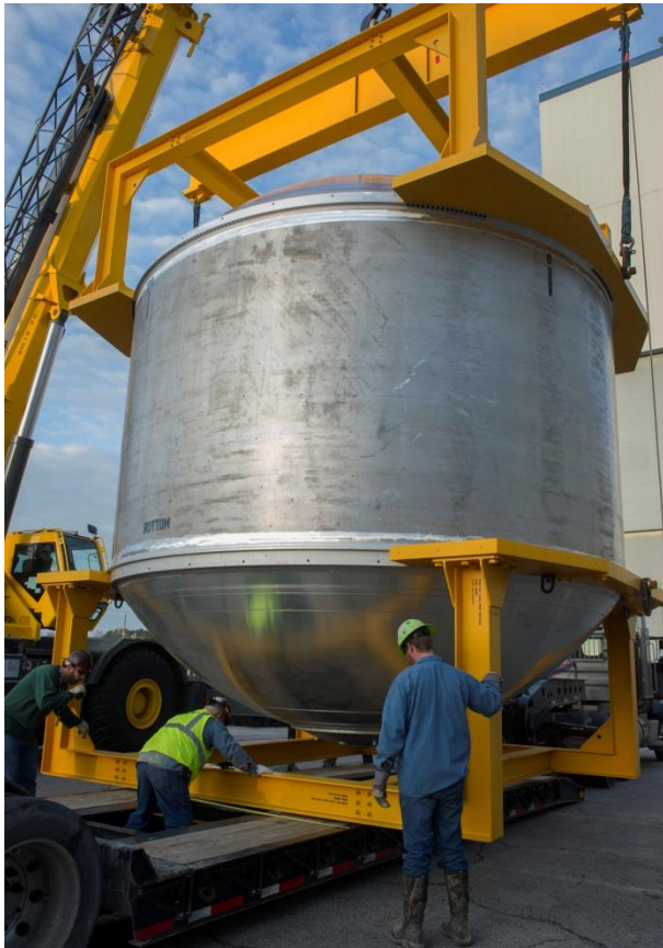
Fig. 21. Moving the completed tank across MSFC to the river.
