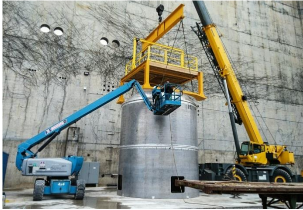
Fig. 25. Placing the integrated test article on the test pad.
