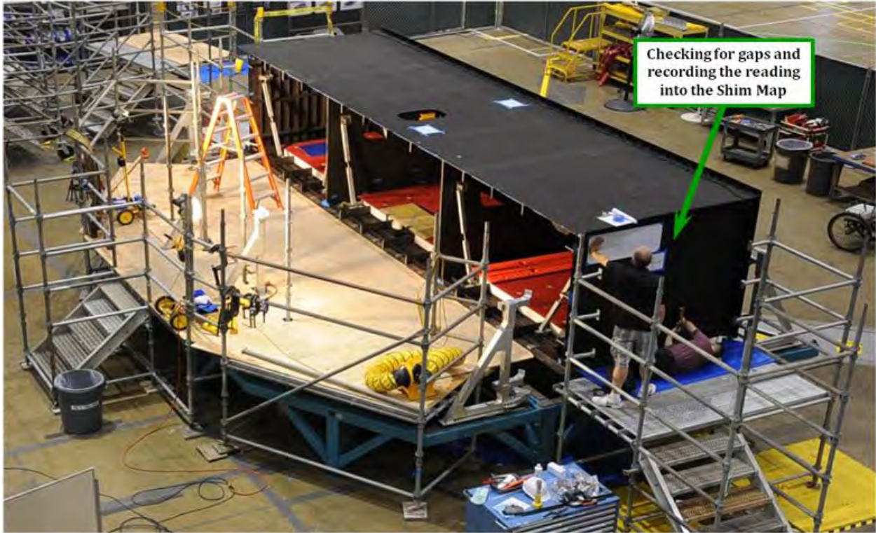
Figure 6-40. Upper Section—Checking for Gaps and Recording Them Into the Shim Map
