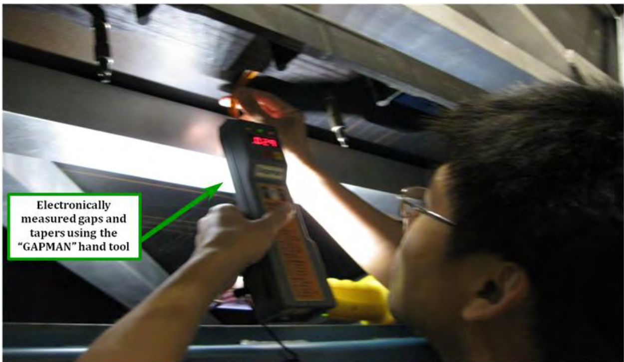
Figure 6-41. Using the GAPMAN Device to Measure Gaps and Tapers
