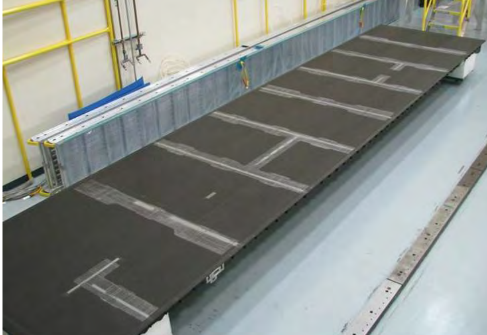
Figure B-11. Bonding Surfaces Were Prepared for Repair Patches
