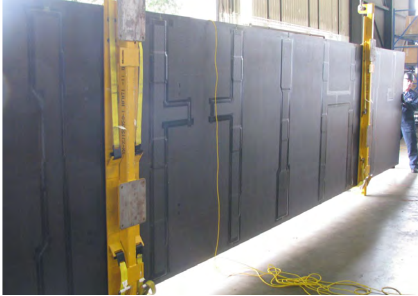
Figure B-15. Completed Bonded Repair Patches on Crown Panel OML
