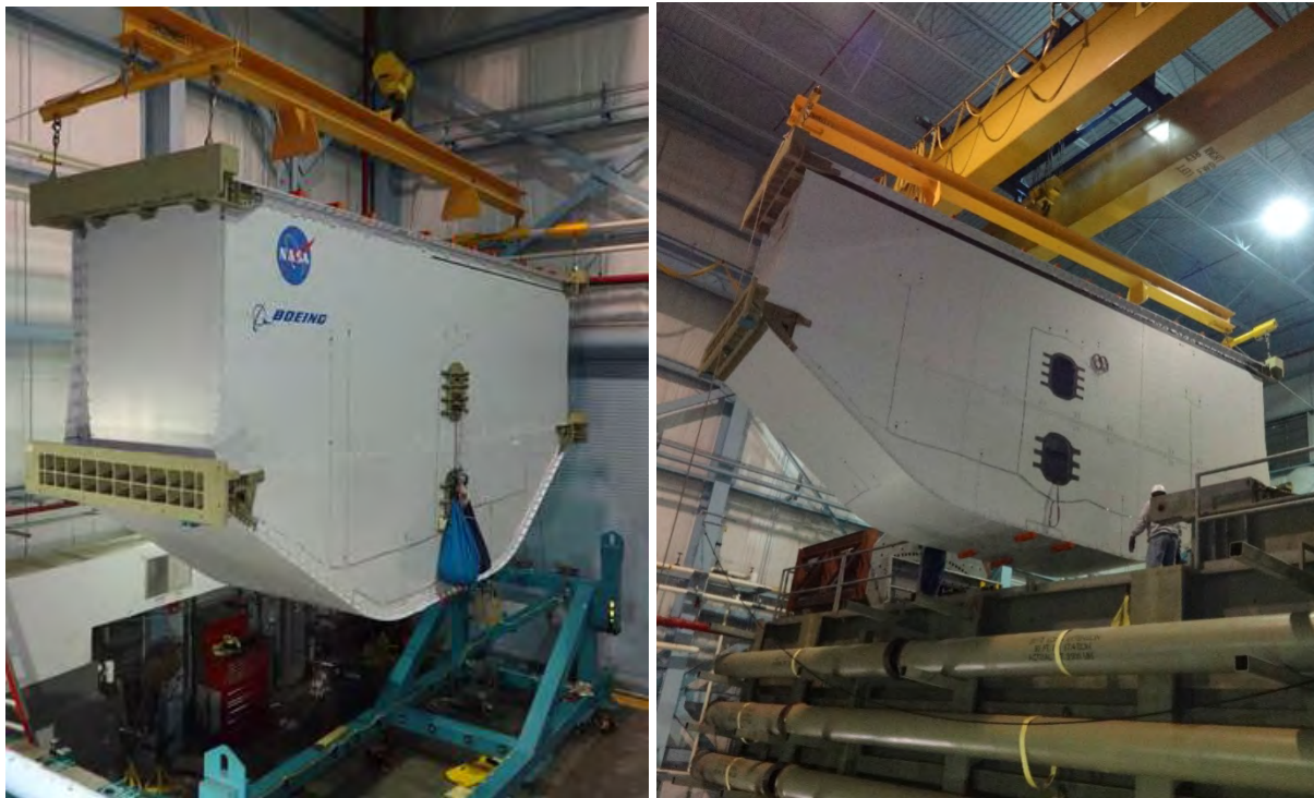
Figure 7-13. Lifting the MBB into the COLTS Test Cell
