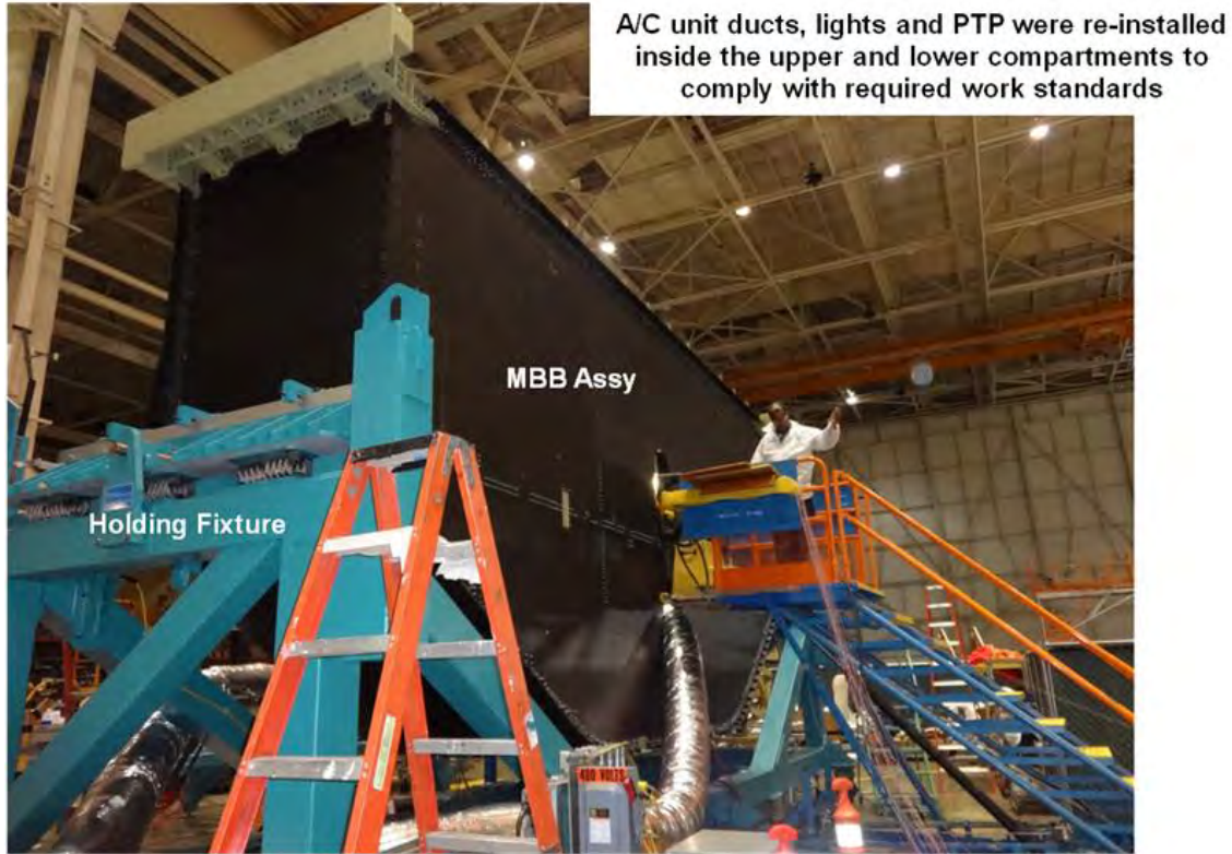
Figure 6-70. Multi-bay Box Assembly on the Holding Fixture
