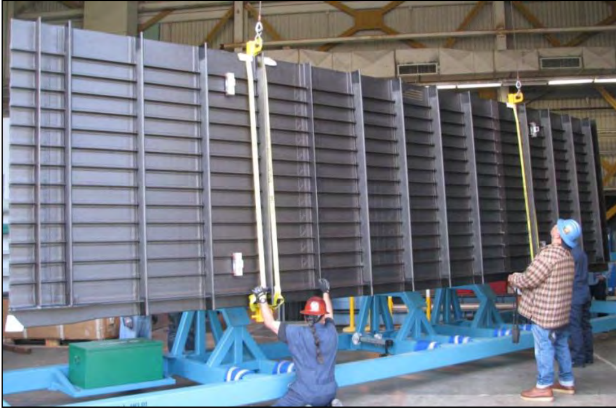
Figure 6-29. Upper Bulkhead Panel Loaded Onto Transport Dolly for Shipment
