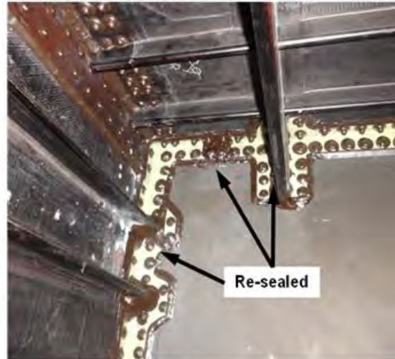
Upper Center Rib after fixing the leak path
