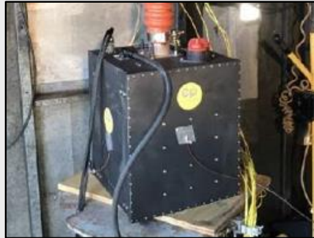
X-57 Battery Module (¼ Pack) before Short Circuit Test
