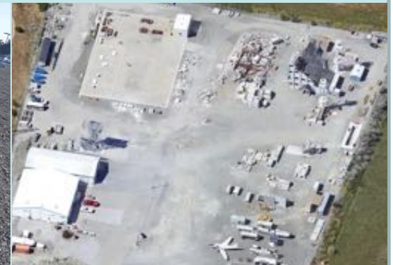
Ames DART Facility
