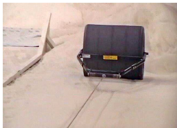
Figure 15.—Soil compacted with a 24-in. lawn roller pulled down the test lane via a mechanical winch.
