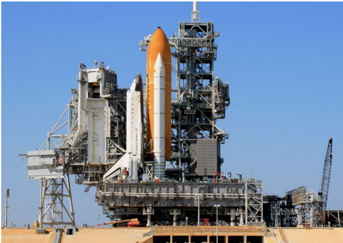
Figure 9. Space Shuttle Launch Structures. (Right) Early two-stage, fully reusable Shuttle ground system architectural concept using Saturn-era Mobile Launcher and umbilical tower. (Left) Actual Shuttle rollout configuration. (Bottom) Space Shuttle launch pad configuration with fixed Pad structures.
