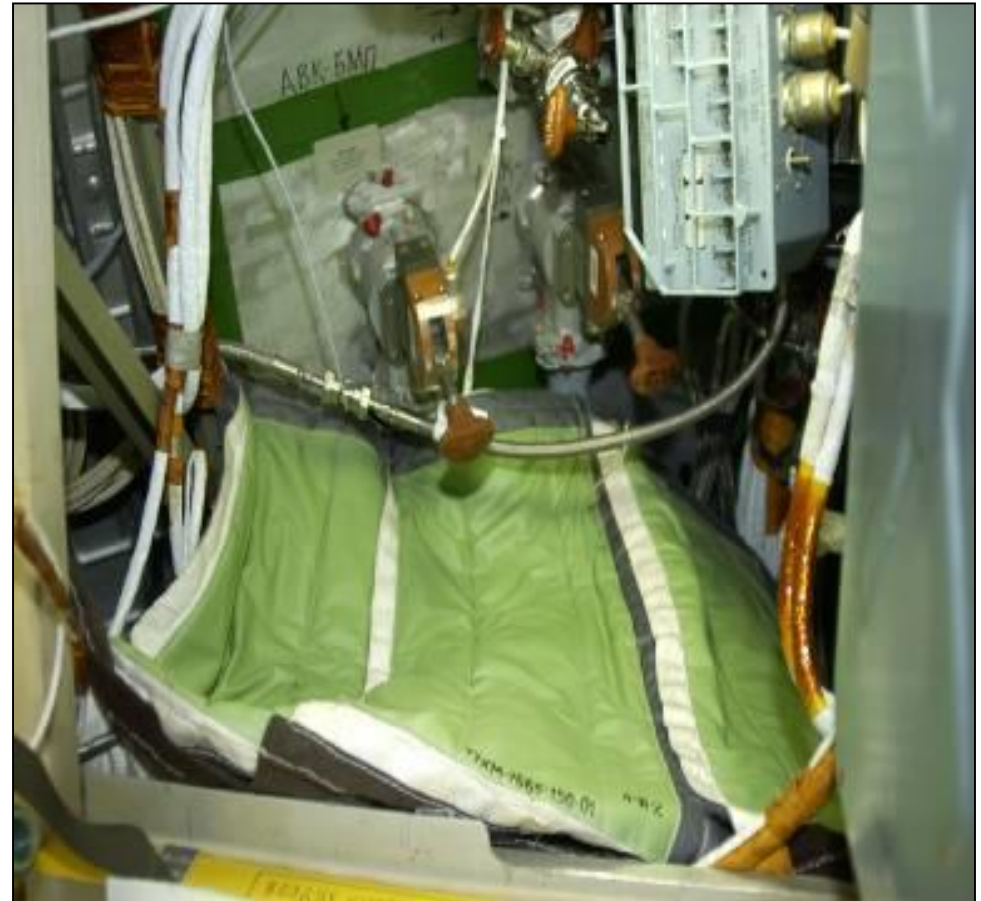
Upon crew initiative, additional soundproofing device installed
