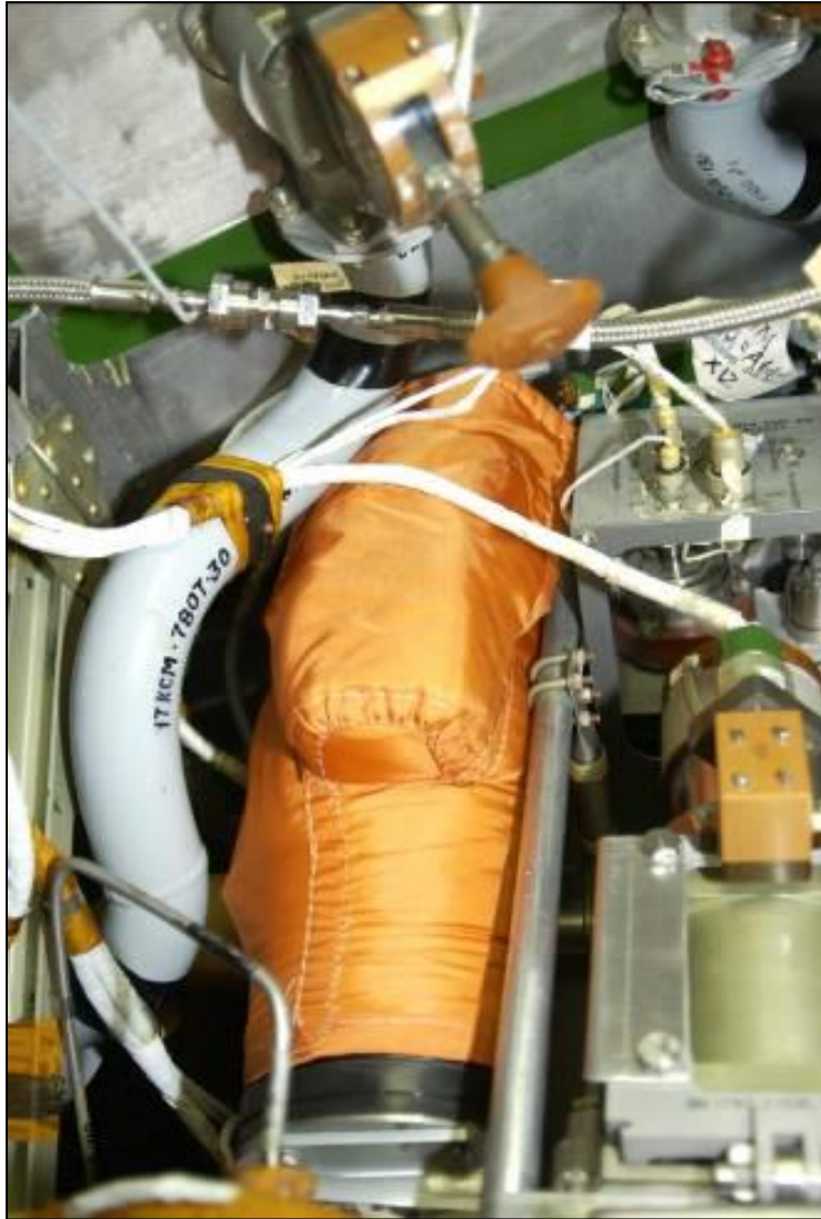
Adapter, shock absorber, and soft soundproof cover installed
