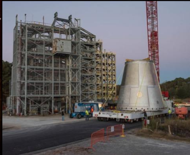
Structural testing at Marshall
