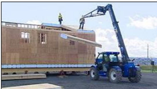
Canadian northern home construction
