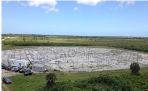
Figure 1. Aerial view of NASA KSC TDRWP. System electronics are housed in trailer on the bottom left of photo.
