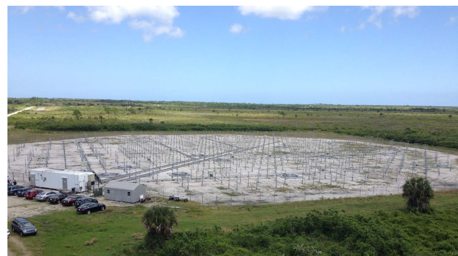
Figure 1. Aerial view of KSC TDRWP. System electronics are housed in trailer.
