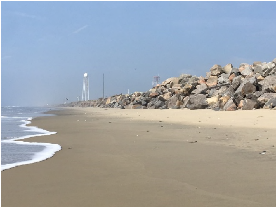
Figure 4- 6: Rock seawall at Wallops Island. Photo taken by author June 2017.
