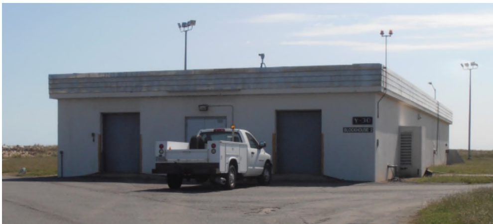
Figure 5- 2: Building Y-30 at Wallops Island. Photo taken by author May 2017.
