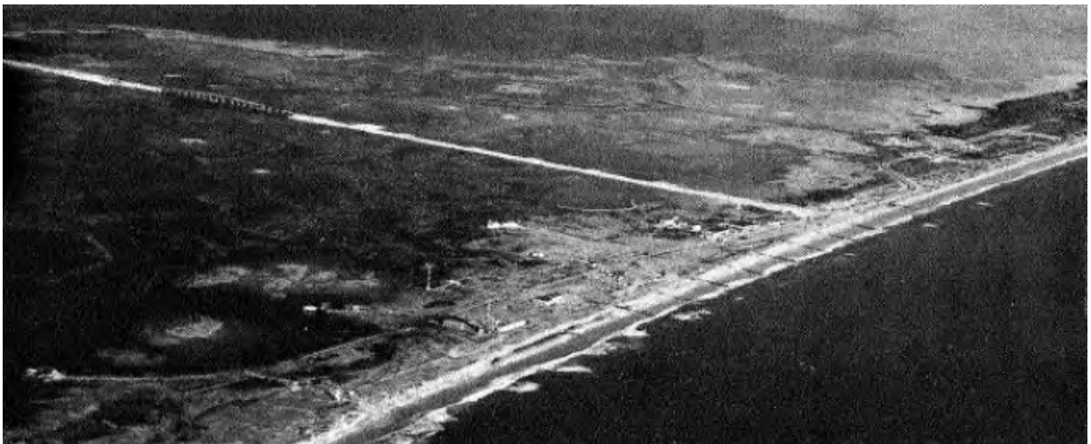
Figure 4- 3: Wooden groins at Wallops Island 1959. (King Jr., Ward, Williams, & Hudgins, 2010)
