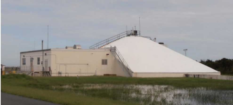
Figure 5- 3: Building W-20 at Wallops Island. Photo taken by author May 2017.
