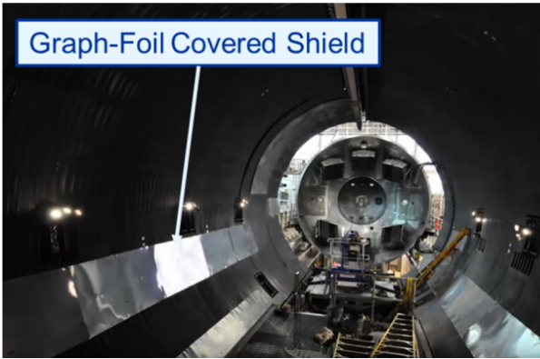
Figure 4.—VF-6 during installation of Grafoil® shielding.
