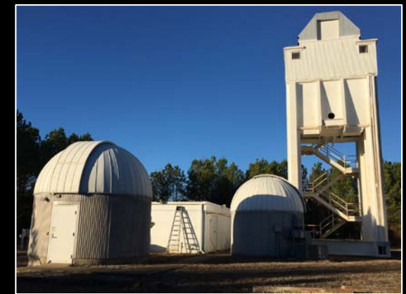
Observing facility at MSFC, operational from May 2006-present: Two observatory domes, a 15 meter (50 ft) tower with a roll-off roof, and an operations center with laboratory space.
