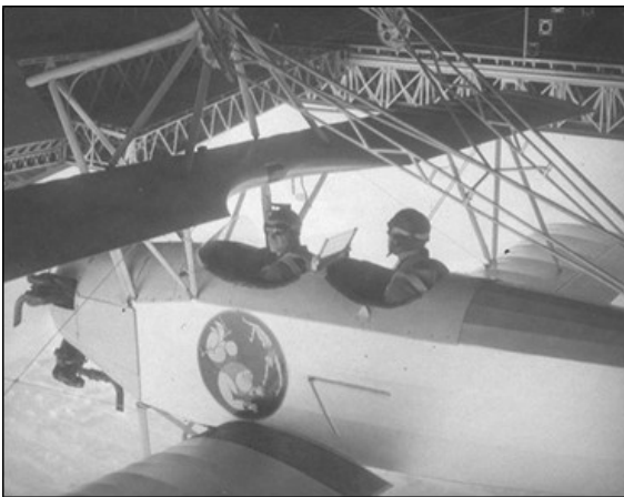
Plane hauled into USS Macon hangar
