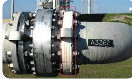
KSC and University of Central Florida researchers developed a color-changing tape that could detect hydrogen leaks.
