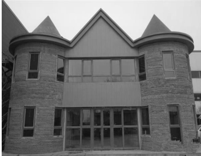
Figure 1: 3-D Printed Villa – China
