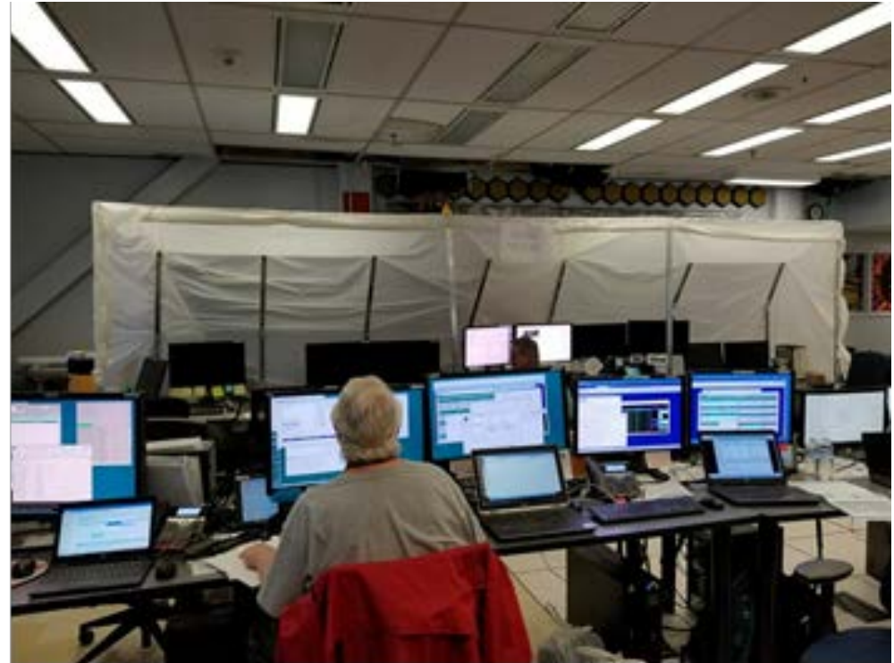
Plastic Sheeting installed to Protect control computers and data stations
