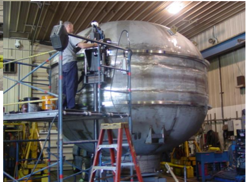
Machining Tank Flanges
