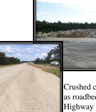
Crushed concrete utilized as roadbed for local Highway 607 expansion
