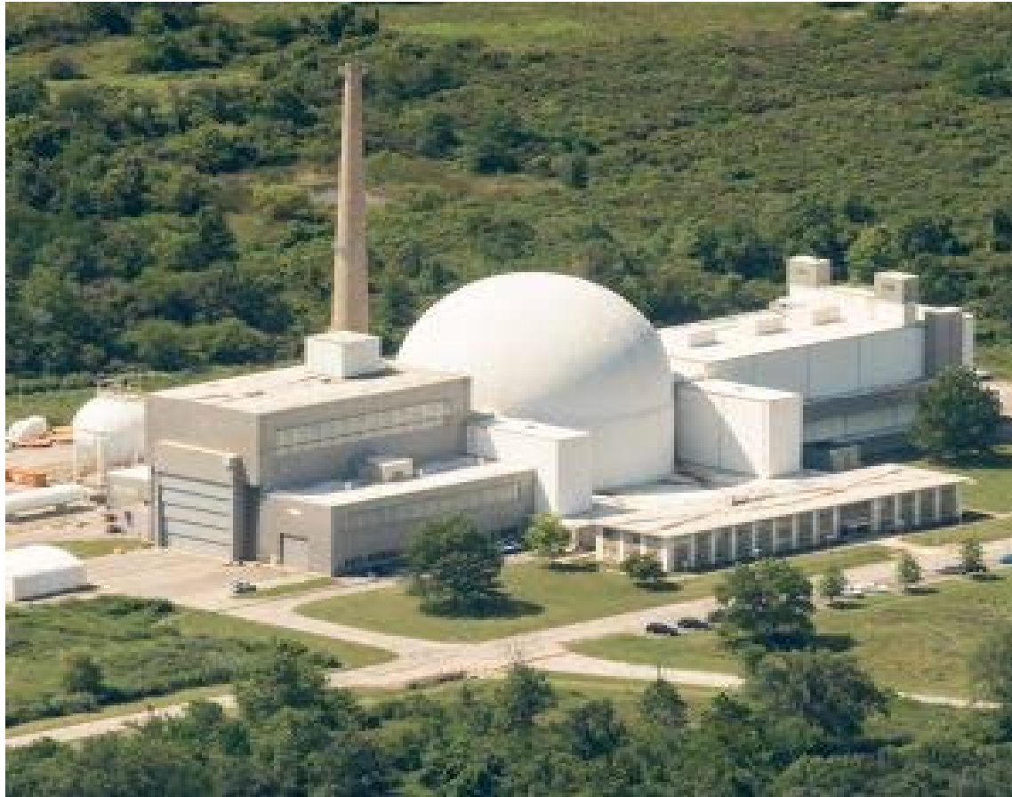
Figure 9: Space Environments Complex (SEC) aerial view.
