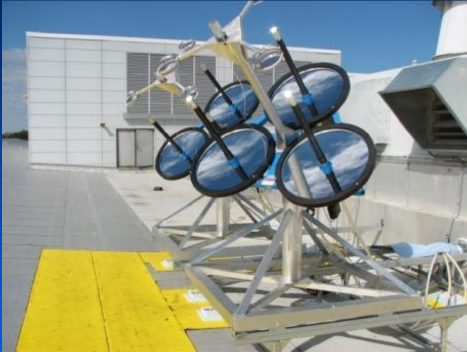
2 m 2 of collectors on solar tracking drive (SLSL Bldg, NASA KSC)
