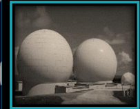
Guam Remote Ground Terminal
