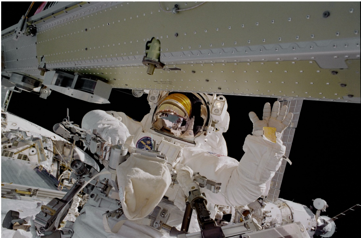
Figure 55.—Astronaut Carlos Noriega during an Extravehicular Activity to repair 2B tension system. Array blanket box is shown at top of image with tensioning spools are on left (sts097-376-009).
