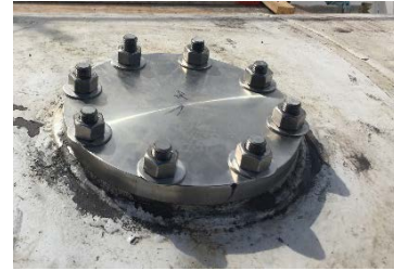
Figure 4, New Pearlite Fill Flange Configuration
