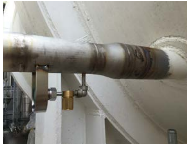
Figure 1, Typical Thermocouple Vacuum Tube Installation
