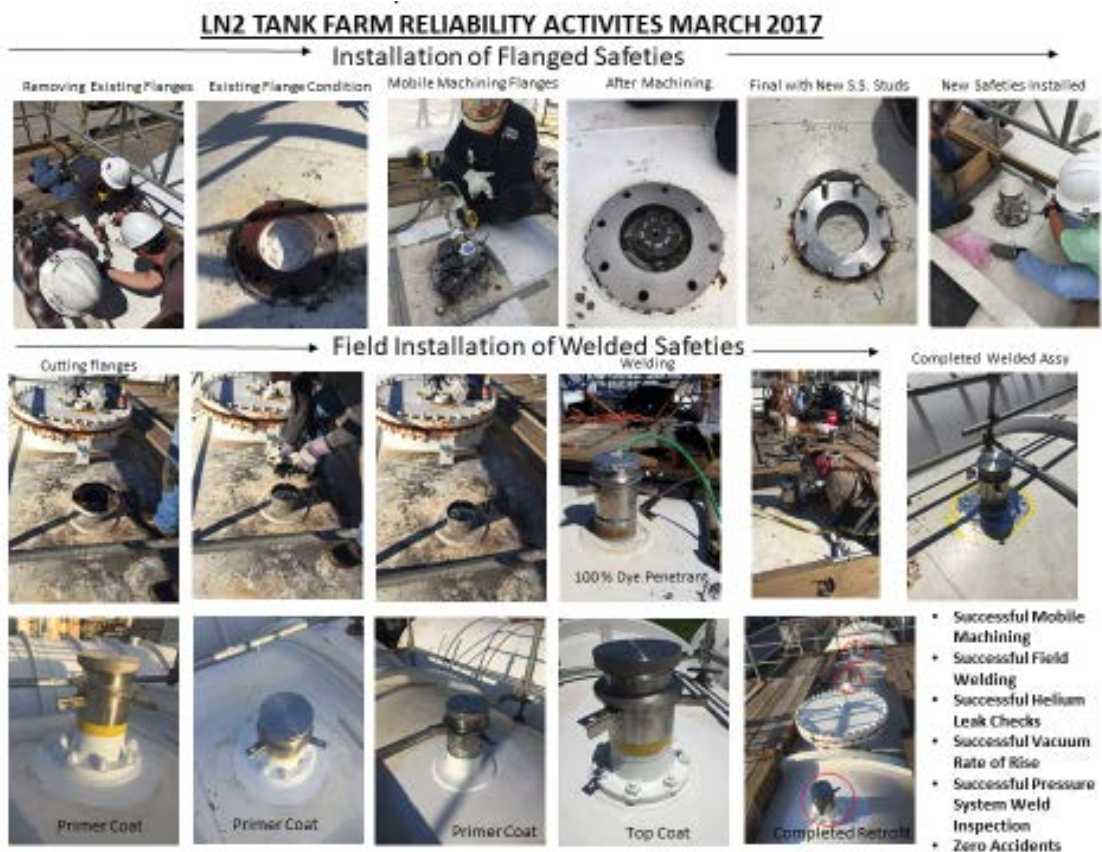
Figure 7, Phase 2 Project Photograph Summary
