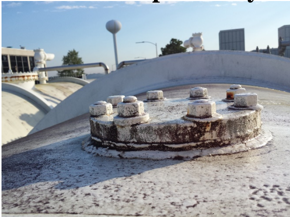
Pearlite Fill Flange, Carbon Steel
