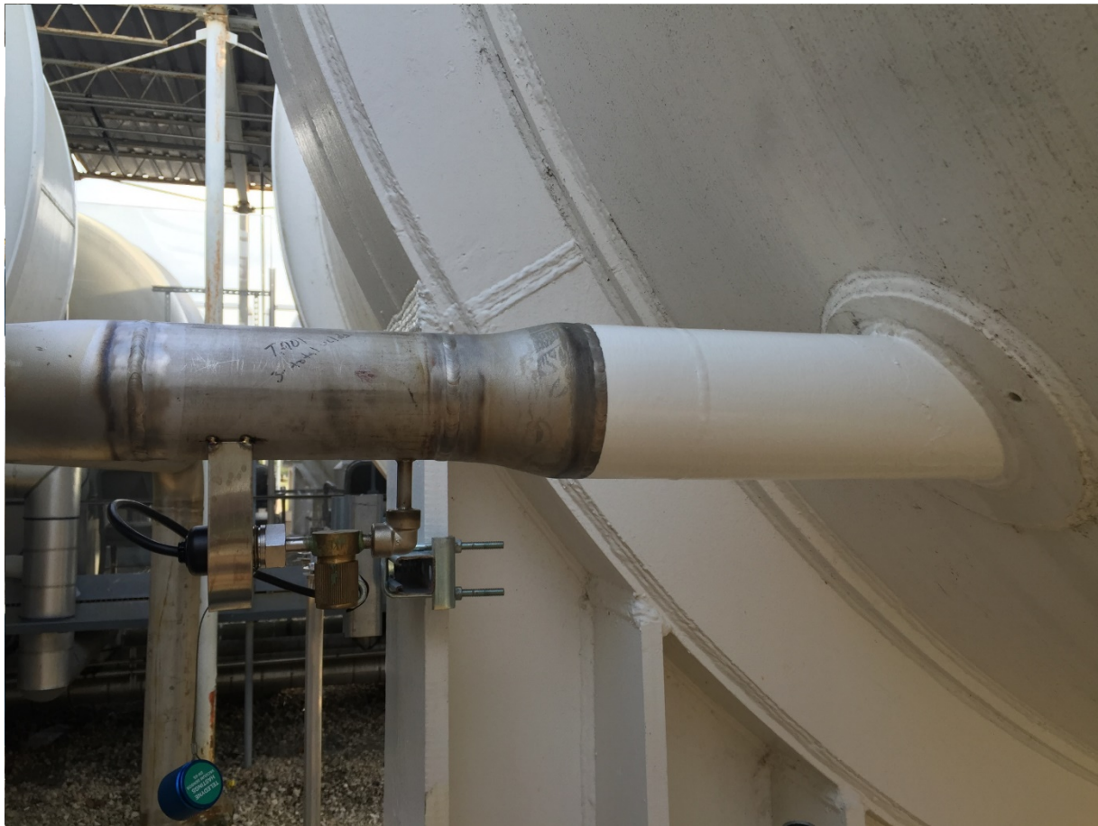
NEW INSTALLED PIPING WITH COATING
