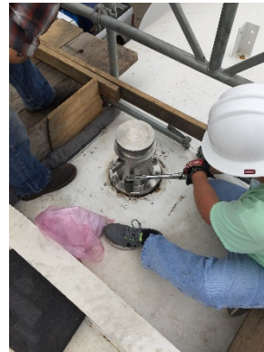
New Safeties Installed
