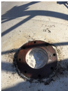
Existing Flange Condition
