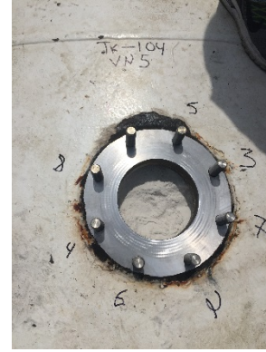
Final with New S.S. Studs
