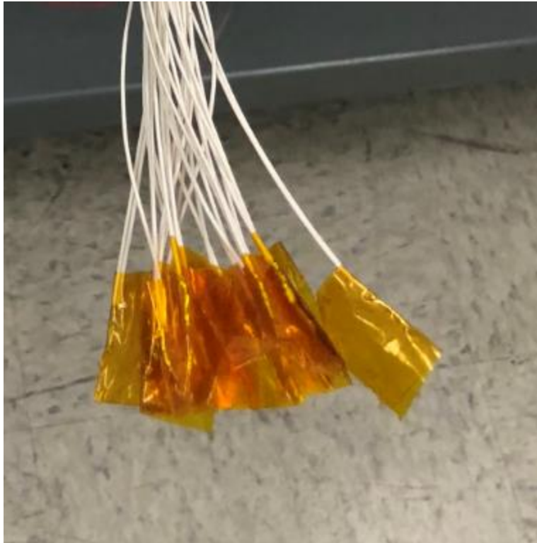
Figure B.2-9. Soldered Wire Ends covered in Kapton® Tape
