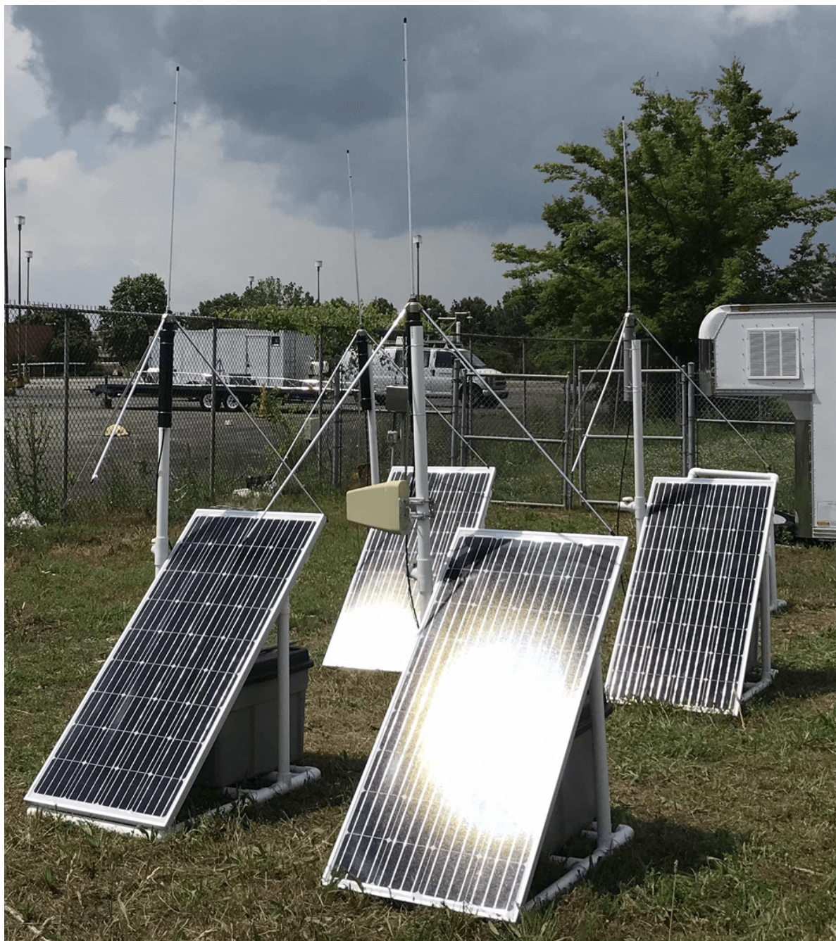
Figure 1. Refurbished LMA stations at the NSSTC, prior to shipping.
