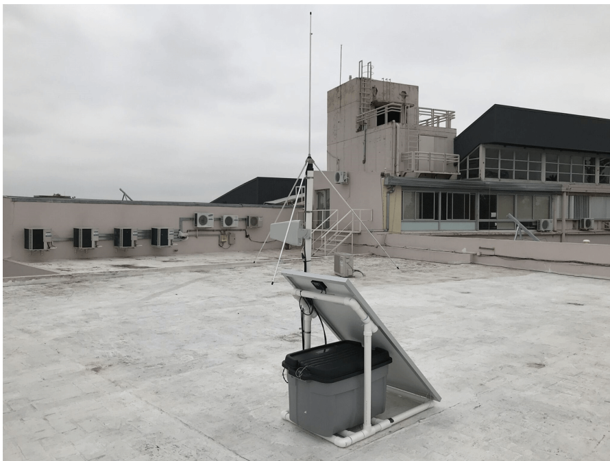
Figure 4. LMA station on top of roof at UNC.
