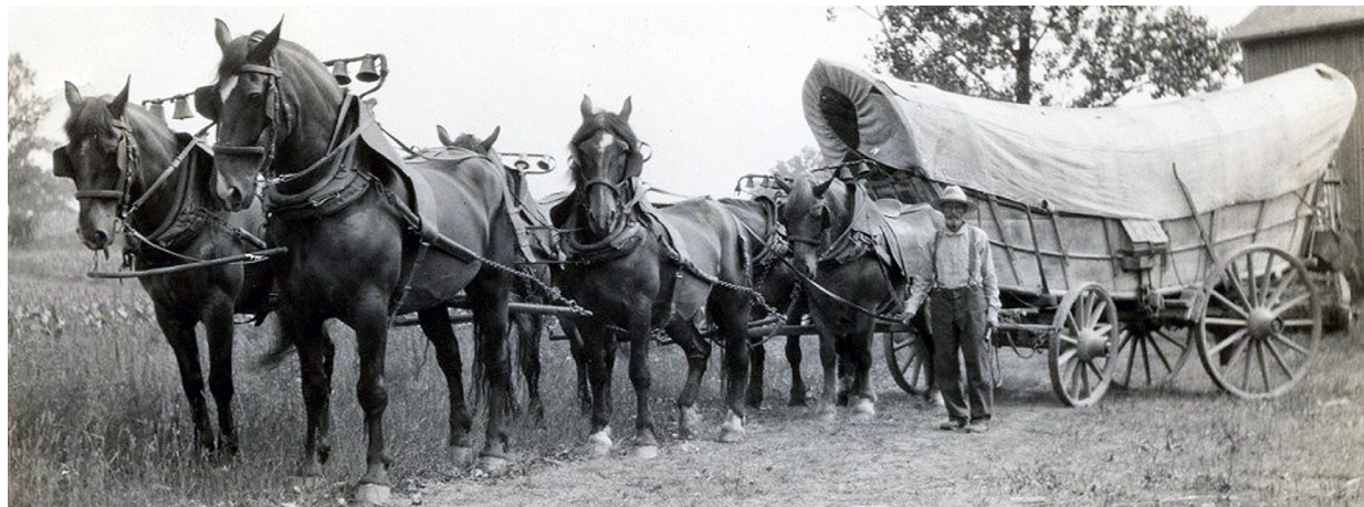
Figure 17.—Conestoga wagons, the “ships of inland commerce,” were used from 1700s to early 1900s to transport settlers, farm produce, and freight across Pennsylvania and neighboring states (image ca. 1910). Courtesy of Landis Valley Village & Farm Museum, Pennsylvania Historical Museum Commission.
